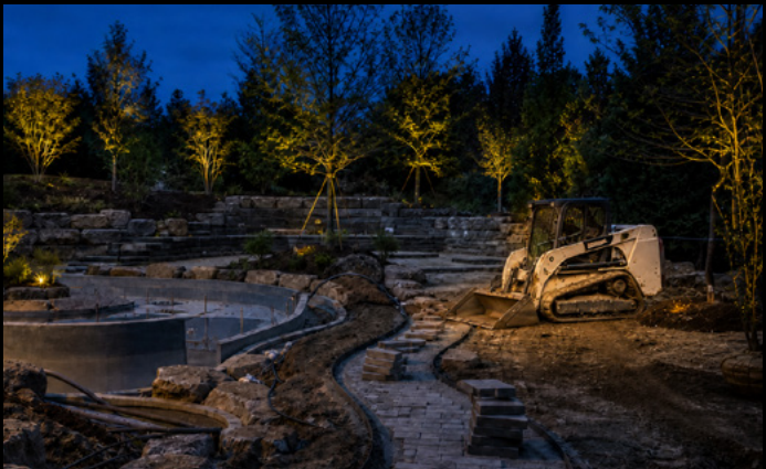
Retrofit and renovation
